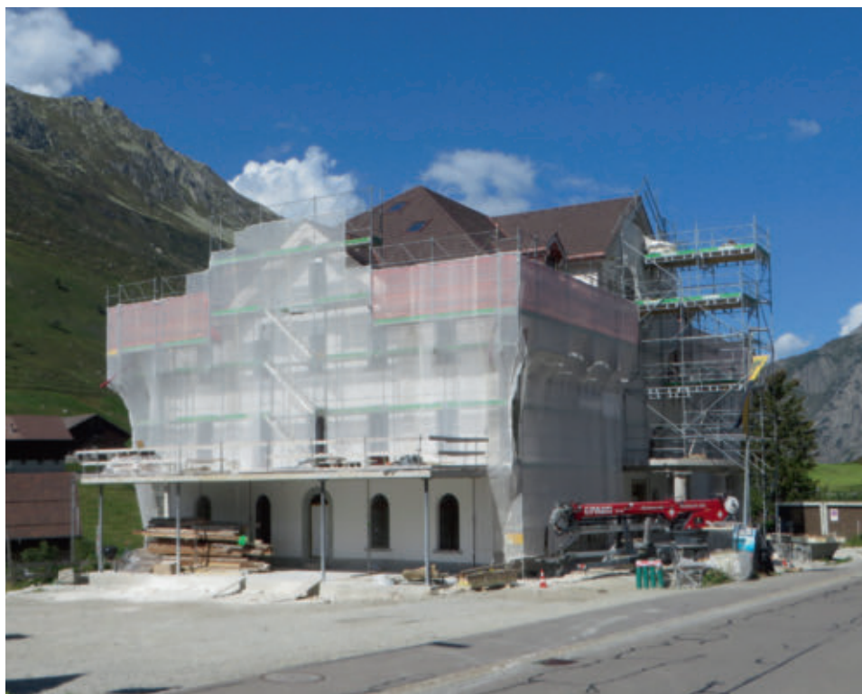
Renovation des Meyerhofs in Hospental am 5. September 2021.
